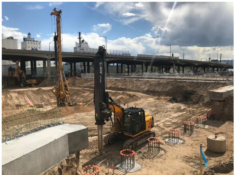
Construction of Monroe Street Bridge
