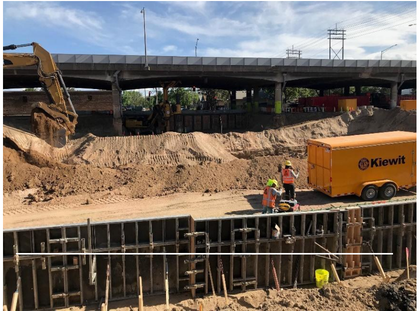
Looking south at the Columbine Street bridge abutment
