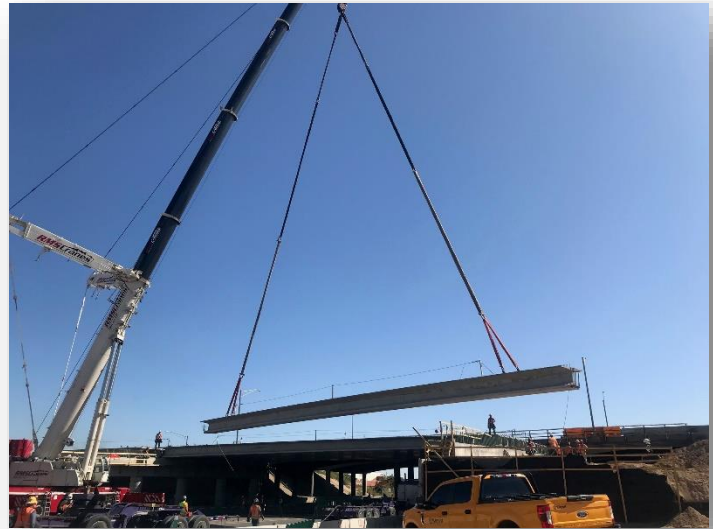
Girder set at Colorado Boulevard Bridge
