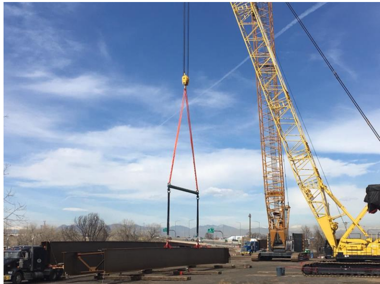
I-270 flyover girders getting ready to be set
