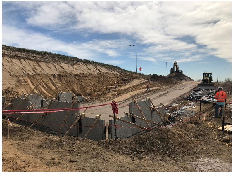
Construction of the bridge abutment for the I-270 flyover
